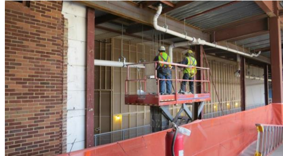
Figure 2: Existing S. Wall Demolition Courtesy of Mortenson Construction
